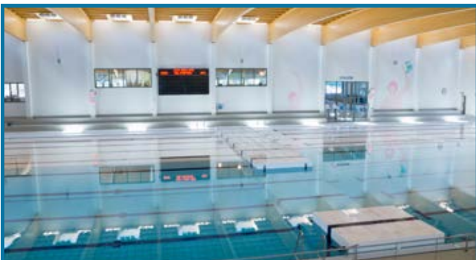
S&R Olympia Brugge, Belgium: Movable floor and Vertical bulkhead 3-section
