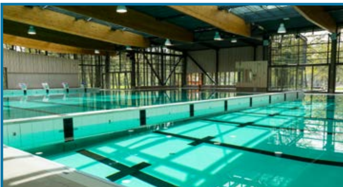
Warande recreatieoord Oosterhout, the Netherlands: Movable floor with integrated steps, bulkhead, Disabled platf.
