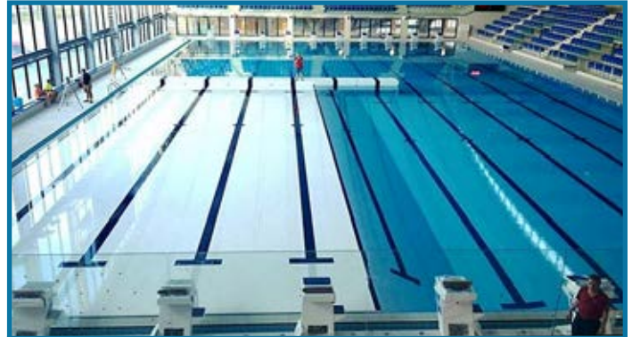
Aquacomplex Lublin, Poland: Movable duo-floor and hinged bulkhead
