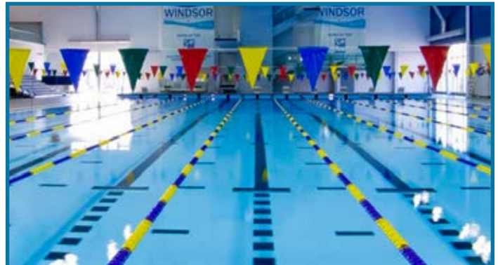
Windsor Aquatic Centre, Canada: Movable floor
